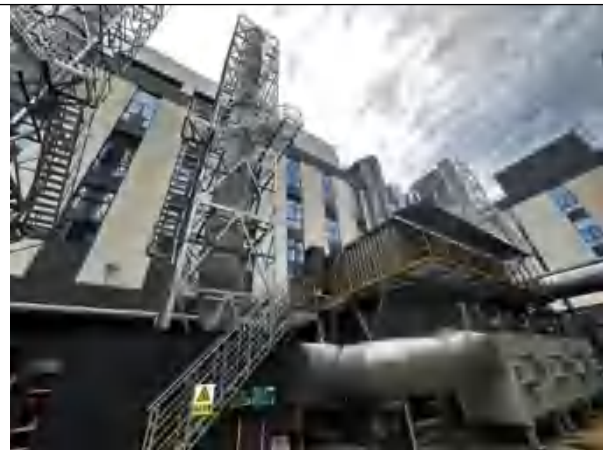
DA009B 线 RTO 排气筒及走梯
